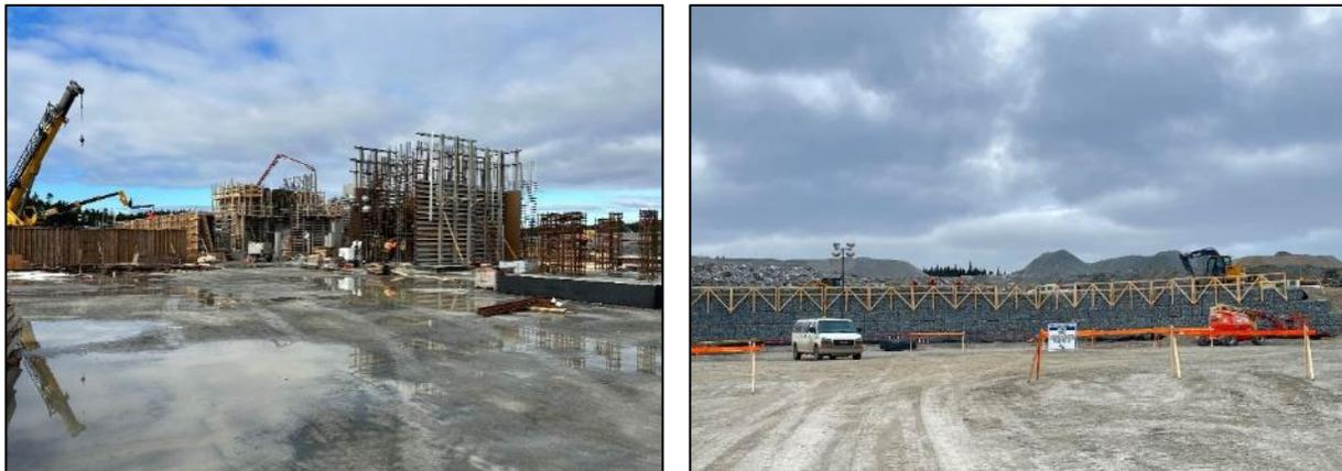
*Figure 3: Concrete Pedestals for the SAG and Ball Mills and Grinding Building Steel Work (left). Gabion Basket Installation for MSE Wall at Crusher Location (right). October 2023*
