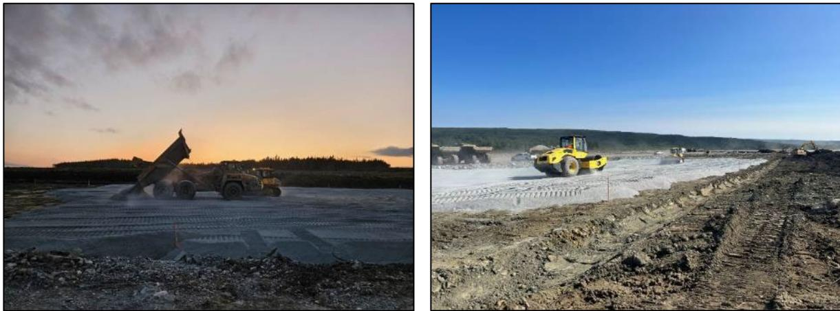
*Figure 4: Construction of the TMF. Spreading Filter Layers for Geomembrane Liner Placement. September 2023*
