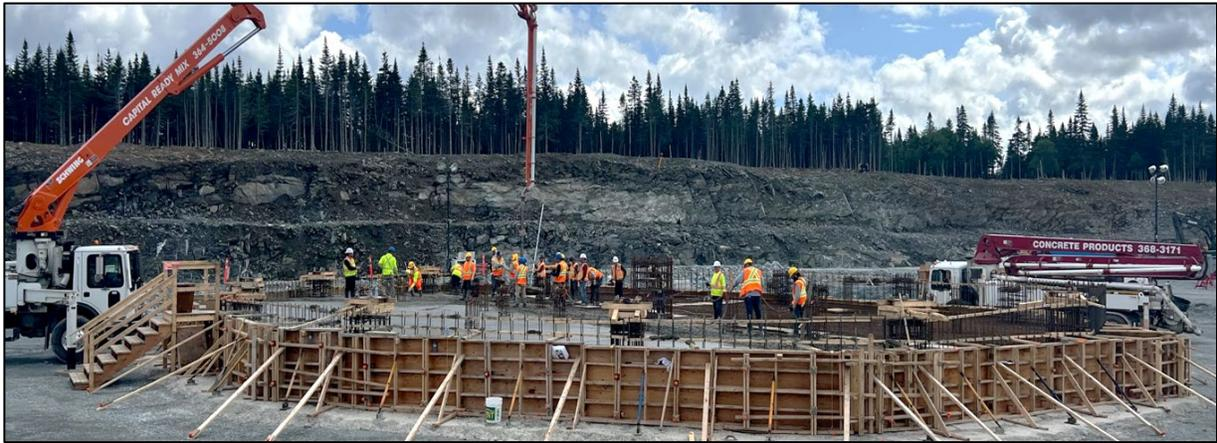
Figure 3: Concrete Slab and Formwork, SAG/Ball Mill (top left), Transformer Installation (top right), Tailings Thickener Concrete Pour (bottom). All July 2023
