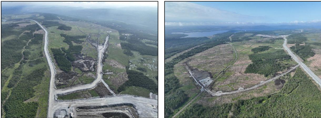
*Figure 5: Construction of the Toe Road for the Tailings Management Facility. Advancement of the construction toe-road from the southwest (left) and northeast (right) simultaneously, July 2023*
