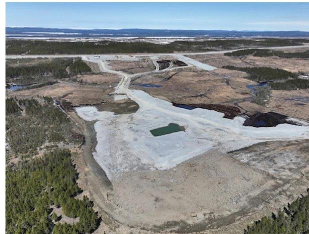
*Civils work underway at the future process plant site. On the left, a NW view showing bedrock blasting on the left and the haul road and Leprechaun Mining pit in the far background. On the right, a NE view showing the haul road and overburden stockpile location in the background. Both photos April 2023.*
