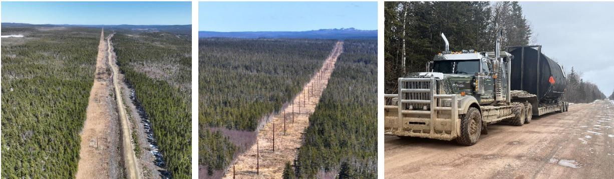
*Left and Middle. Right-of-way clearance and transmission poles on the 44.5 km long powerline route. Right. Shipment of camp water tank by road. Both photos April 2023*
